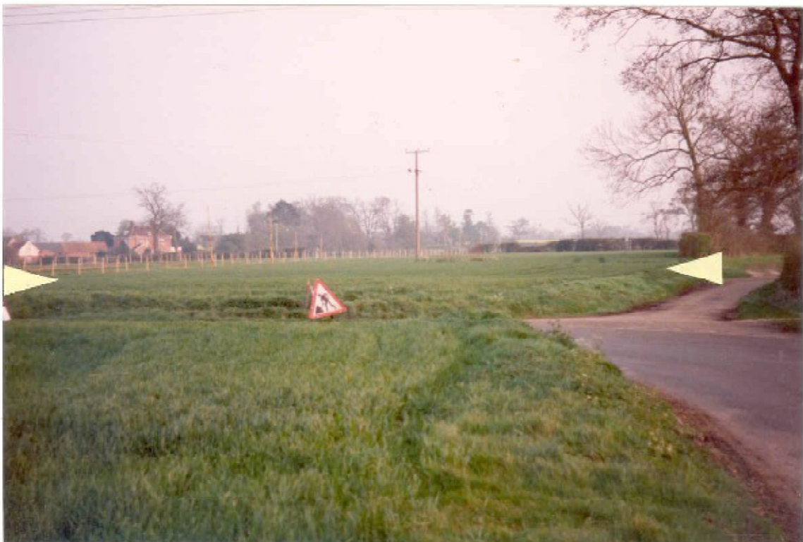
Figure 5.35 Dickleburgh, degraded talus on limes.
