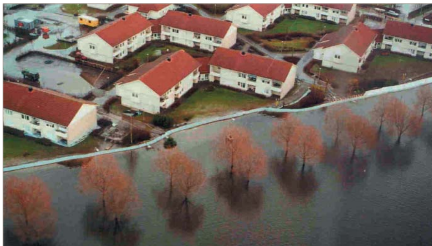
Fig. 3. Temporary/demountable barrier in operation (courtesy Pallet Barrier, Geodesign AB)
