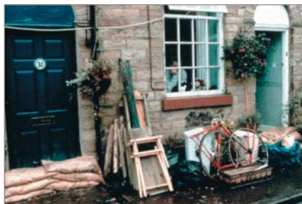
Fig. 1. Sandbag protection to property—indicative of a reactive rather than proactive approach
