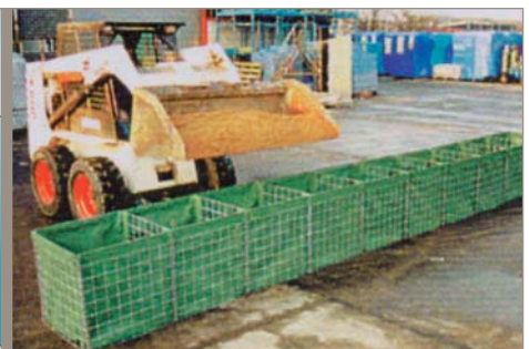
Fig. 8. Temporary barriers can be used to protect a small, otherwise undefended, community
