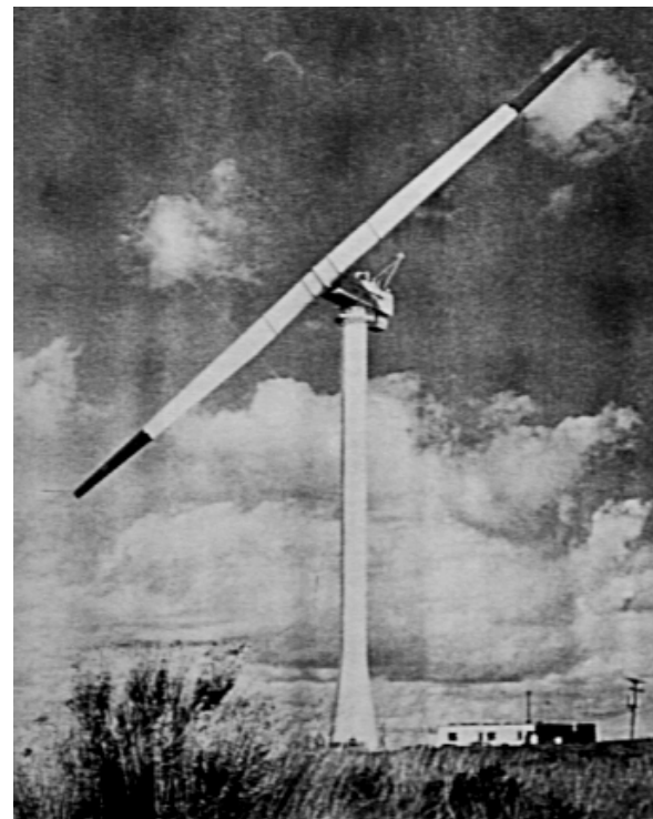
Fig. 16.4 An early 2.5 MW Wind Turbine in Hawaii. The blade diameter is over 90m.
