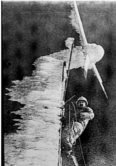
Fig. 16.9 Ice formation on a Wind Turbine
