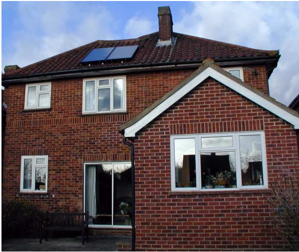
Fig. 15.14 Broadsol installation in Norwich
