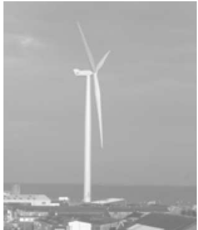
Fig. 16.6 Largest onshore wind turbine (2.75 MW) in UK at Ness Point, Lowestoft, although this will shortly be surpassed with 3MW machines becoming common.
