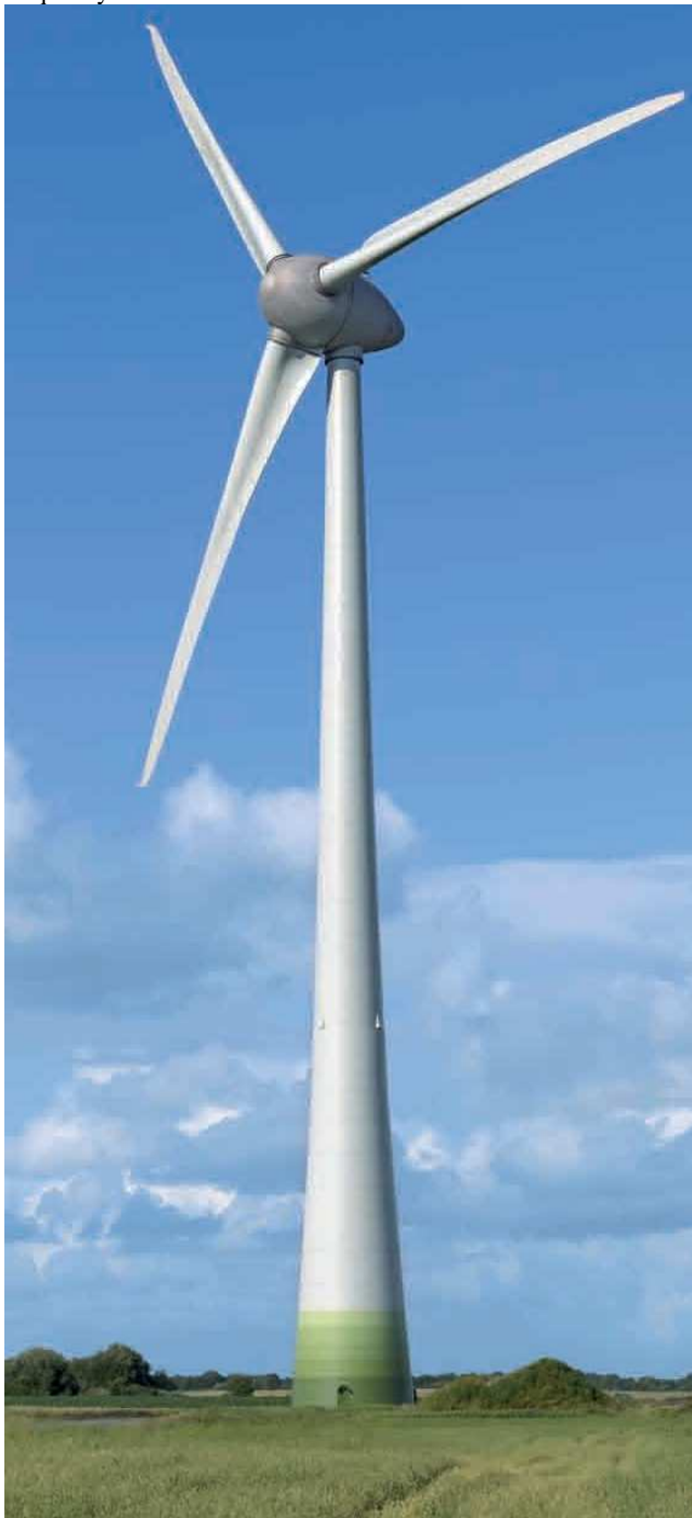
Fig. 16.5 An Enercon E126 wind turbine – the largest yet built with a rated output of 7.5MW, a rotor diameter of 127m and a hub height of 135m.
