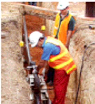
Figure E.1 - HVDC Light land cable burial
