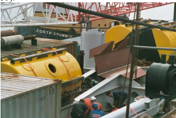
Figure 34: Final Sea Fastenings
