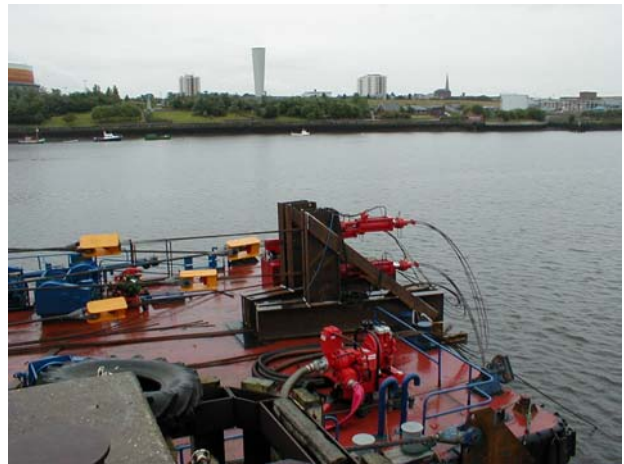
Figure 33: The strand jacks in operation
