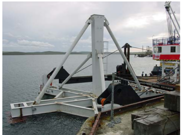
Figure 40: Base assembly suspended from lift beams (photo courtesy of BP)
