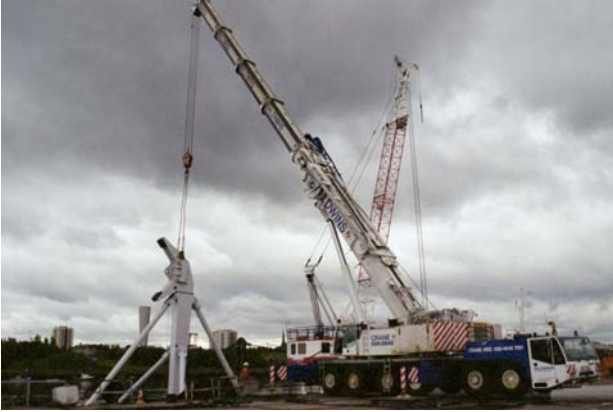
Figure 30: Crane support until strand jacks take up the load
