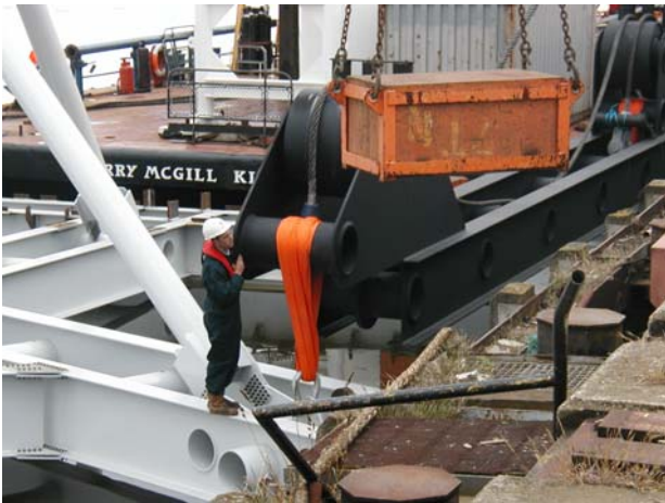
Figure 32: Ballast being loaded onto the Stingray assembly
