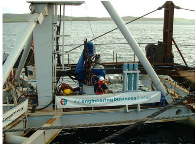
Figure 48: Working on the pod
