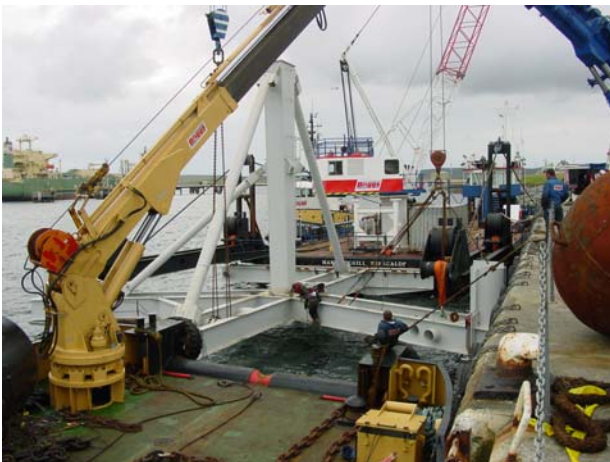
Figure 39: Base assembly suspended from lift beams (photo courtesy of BP)
