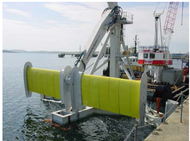
Figure 42: Base assembly suspended from lift beams (photo courtesy of BP)
