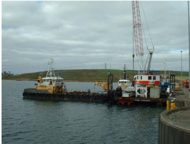
Figure 36: Briggs vessels on Tug Jetty, Sella Ness (Forth Constructor foreground left, Harry McGill with Stingray components foreground right, Forth Drummer background).
