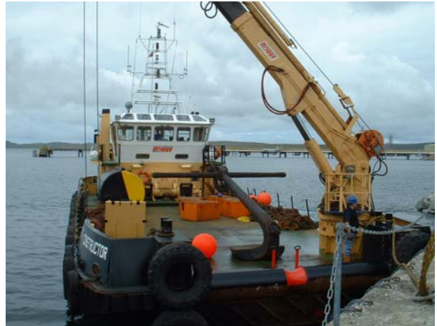
Figure 38: First mooring anchor assembled on Forth Constructor
