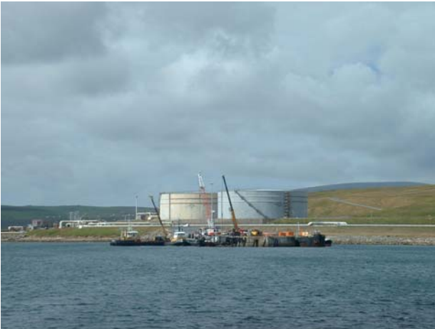
Figure 37: Unloading Stingray components at Construction Jetty
