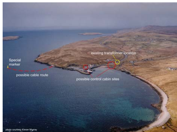
Figure 1: The Site (Photo courtesy Kieren Murray)
