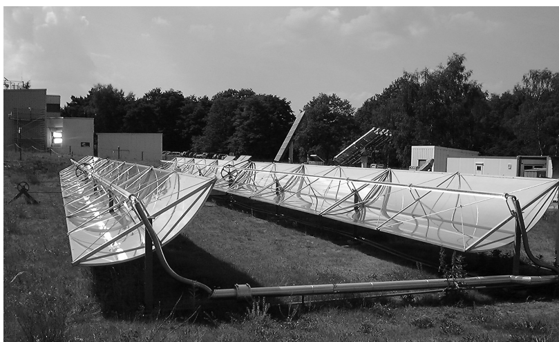
Figure 12: IST-Trough collector at DLR, Cologne
