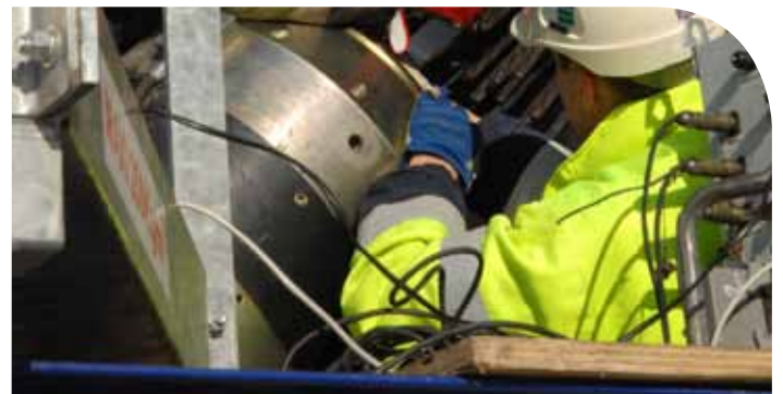
Inner containment pre-stressing activities
