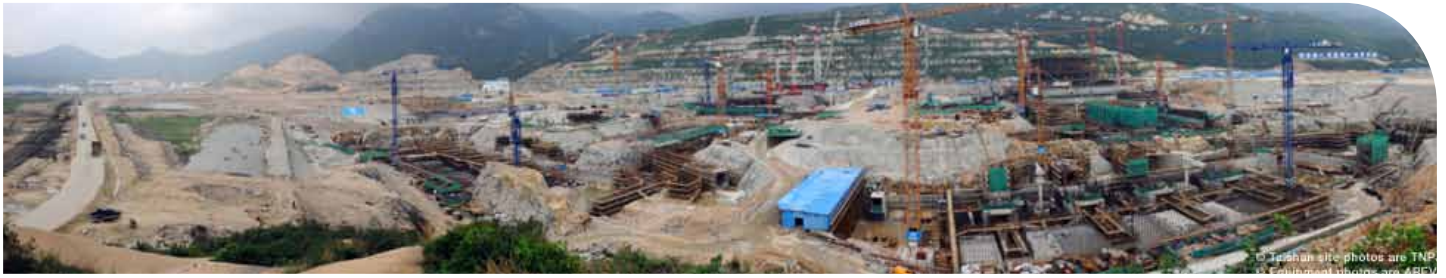
EPR™ projects units 1 & 2 under construction in Taishan, China
