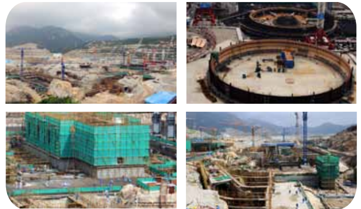
EPR™ reactor unit 2 construction site in Taishan, China
