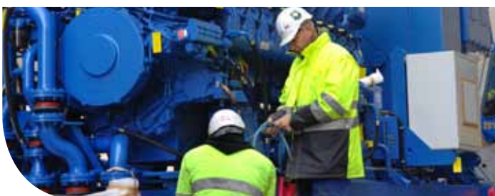
Introduction of the two SBO Diesel Generators into the Diesel Building
