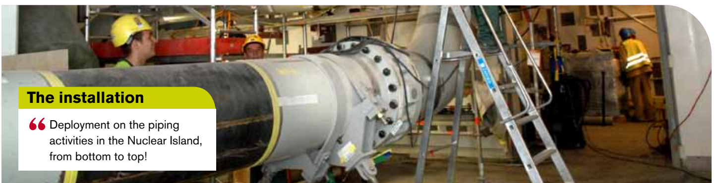
Safeguard Building, Olkiluoto 3, Finland
