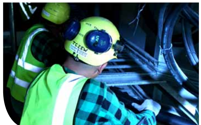
Cable laying, Olkiluoto 3, Finland
