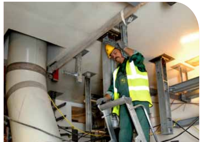
Safeguard Building, Olkiluoto 3, Finland
