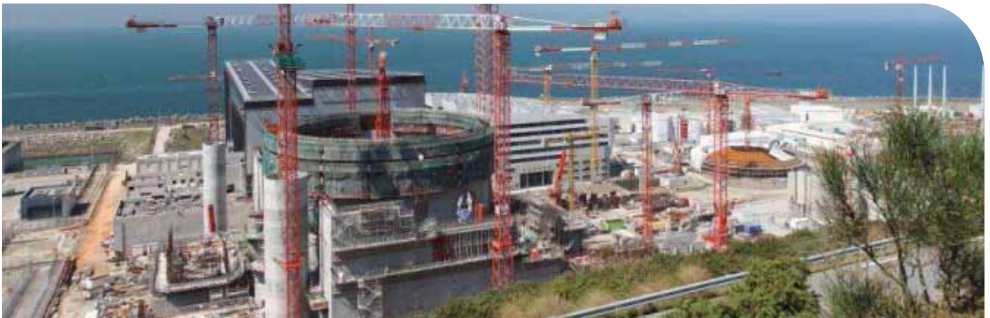
General view of Flamanville 3, France © EDF
