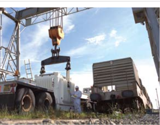
Flask at Wylfa railhead
