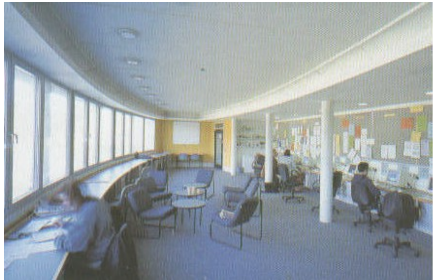
An IT resource room is located directly above the main entrance, and follows the gentle curve of the elevation. Note the row of annular soffit diffusers connecting directly to the exposed Termodeck slabs.
