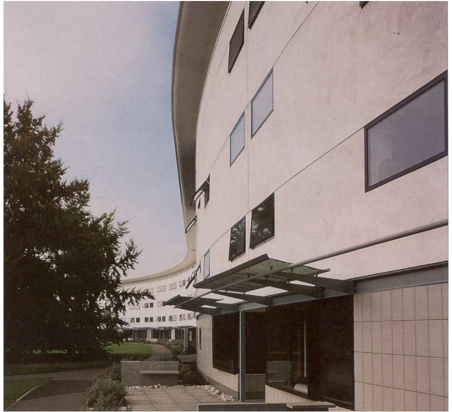
Fig. 2 Part of southern façade, showing external sunshades.
