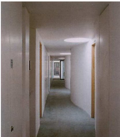
Fig. 3 The third floor access corridor which is daylit via rooflights.
