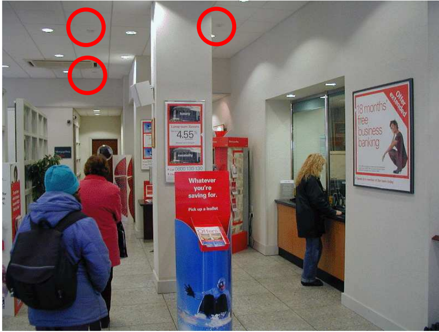
Fig. 47. The main customer area. Notice the spot lights which are unnecessary
