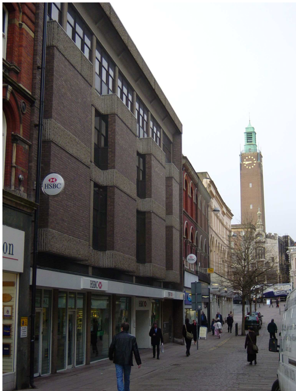
Fig. 20. The exterior of the Norwich Branch in London Street. The top floor is set back from the parapet and not visible in this photograph.
