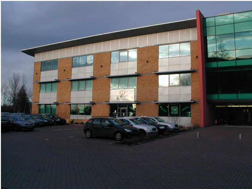
Fig. 8 General View of the southern façade of the building. HSBC occupy the lower two floors. The area to the right is the communal area.
