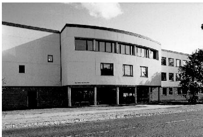
Fig. 5. The Elizabeth Fry Building completed in 1995.
