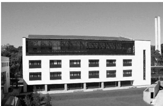
Fig. 7. The ZICER building showing the photovoltaic array on the top floor. On the right the projected performance of the "Termodeck" part of the building compared to the Elizabeth Fry Building.
