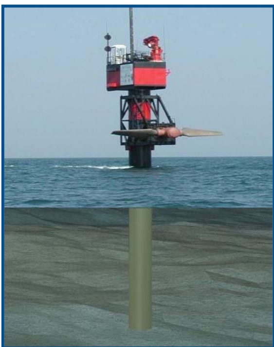
Figure 2: The existing Seaflow tidal stream device in the Bristol Channel Source: Fraenkel, 2003
