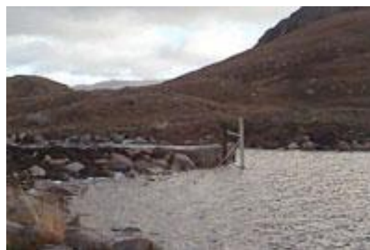
Figure 6: small-scale Hydro scheme, Garbheig, Scotland (Highland Light and Power, 2004)
