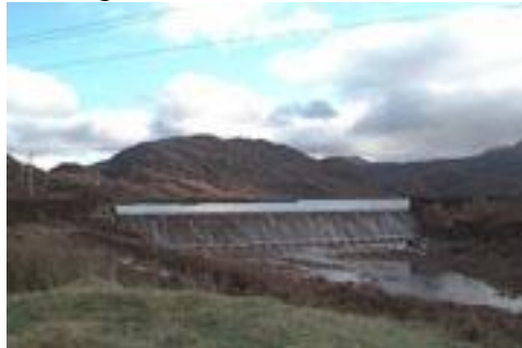
Figure 2: River Kerry Dam (Highland and Light Power, 2004)
