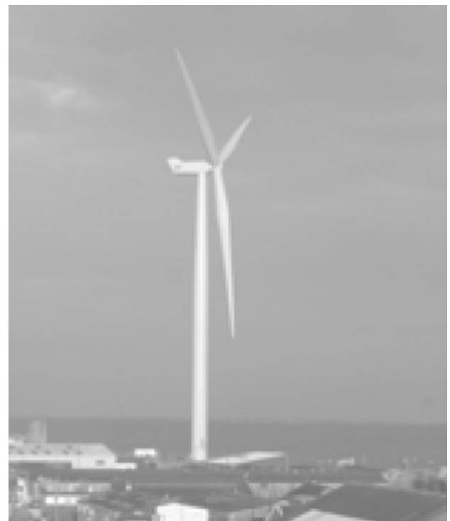
Fig. 24.7 Largest onshore wind turbine (2.75 MW) in UK at Ness Point, Lowestoft
