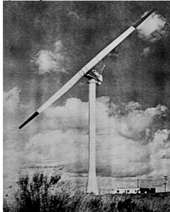
Fig. 24.4 An early 2.5 MW Wind Turbine in Hawaii. The blade diameter is over 90m.
