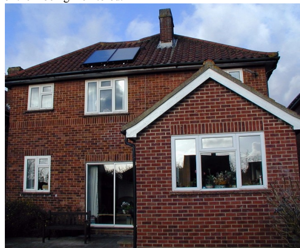
Fig. 23.13 Broadsol installation in Norwich
