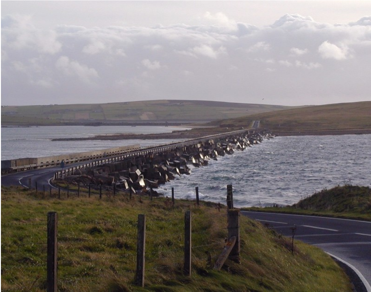
Churchill No 2 Barrier, Orkney. This barrier is 620 m long and was constructed during World War II. There is a difference in tides of 1 hour 40 minutes between the east and west sides of the barrier giving the potential for a tidal barrage without much of the capital costs associated with construction and without most of the environmental problems associated with such barrages.
