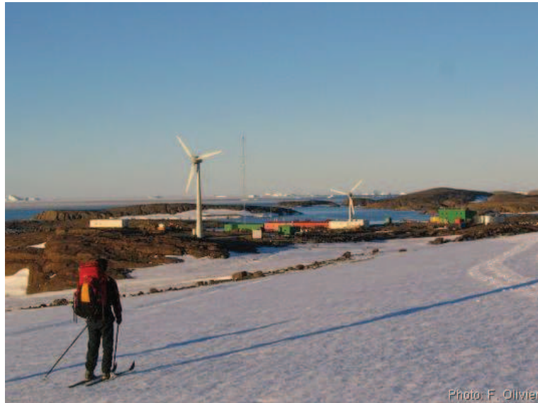
Figure 1.3: The two wind turbines at the Australian Antarctic station Mawson. Photo courtesy of F. Olivier.
